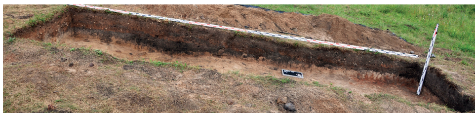
4 pav. Perkasos 1 vietoje nustumtas molio sluoksnis apsaugo kultūrinio sluoksnio likučius. V. Podėno nuotr. Fig. 4. The clay layer, which has been removed at the site of trench 1, is protecting the remnants of the cultural layer.
